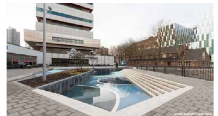
Image 2: Benthemplein square, during monsoon when the square has water collected through the rain water collection from the buildings around and the space transforms into a water body along the steps.
